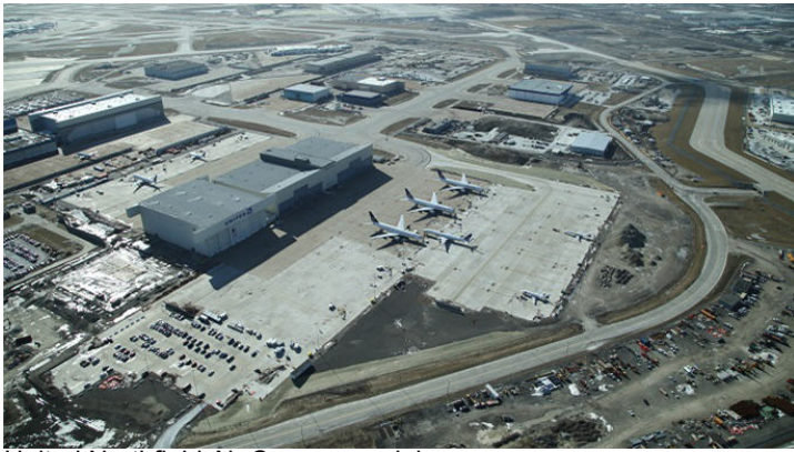
United Northfield Air Campus aerial
