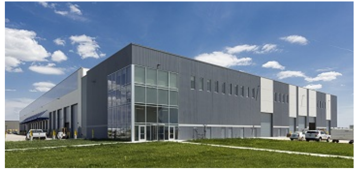
United GEM facility
